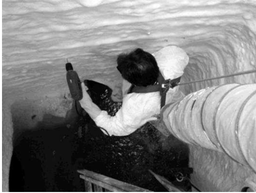
Epoxy-Lining Manhole Repair, St. Thomas
